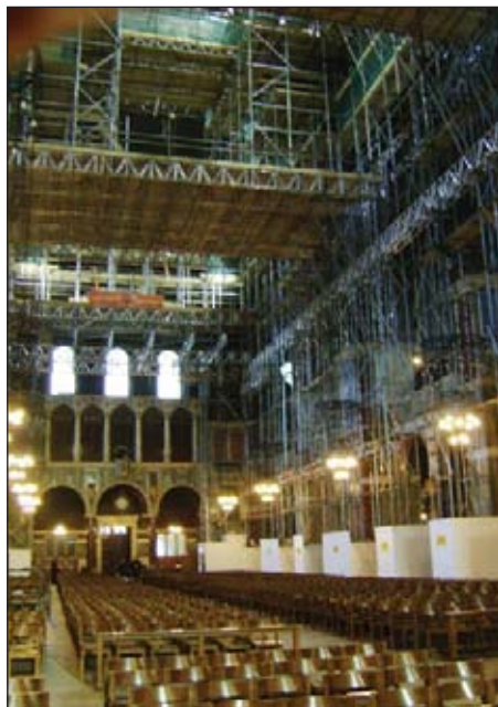
Scaffolding throughout Westminster Cathedral, London
